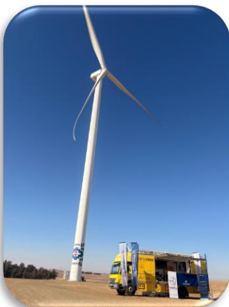
The energyDRIVE bus parked beneath an operating turbine at the Goldwind wind farm.
