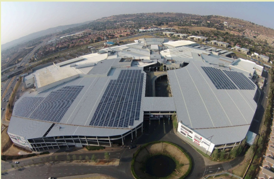
Figure 22: Clearwater Mall 1.5MW of rooftop PV panels – phases 1 and 2
