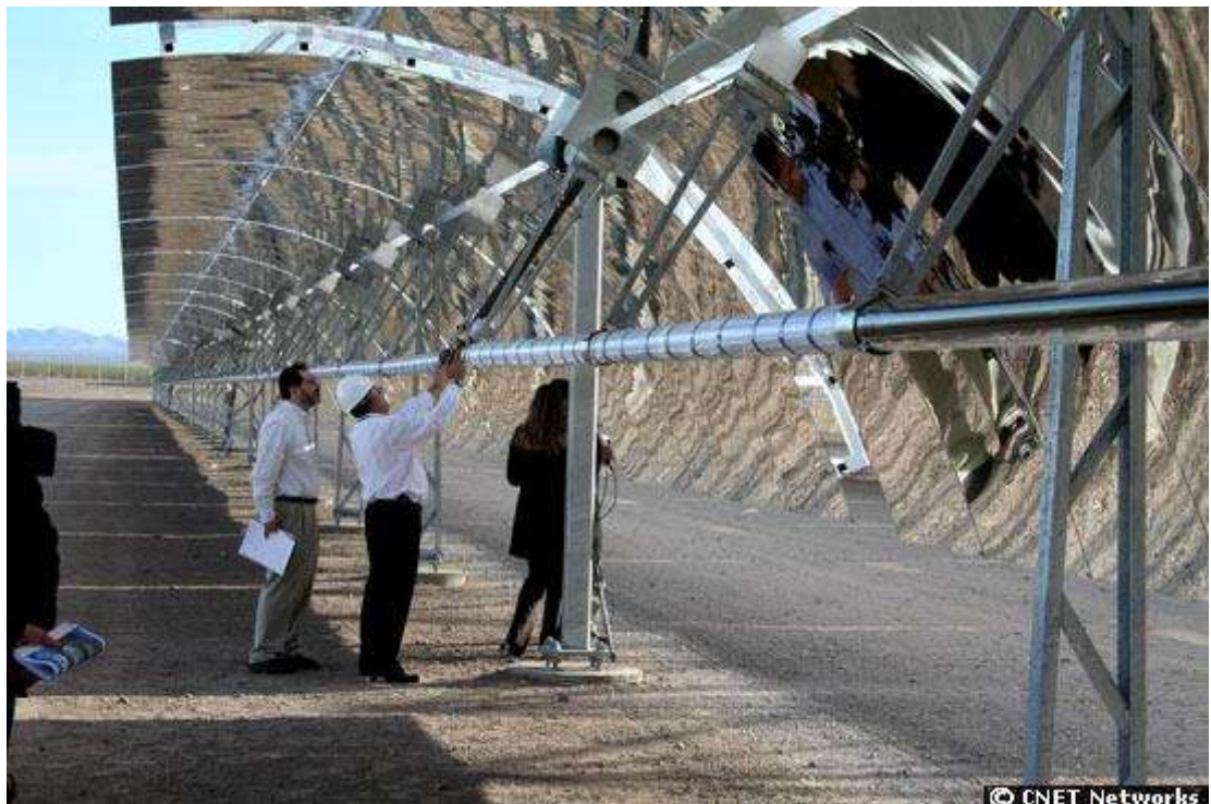
Figure 5-4: Partially stowed trough reflector
