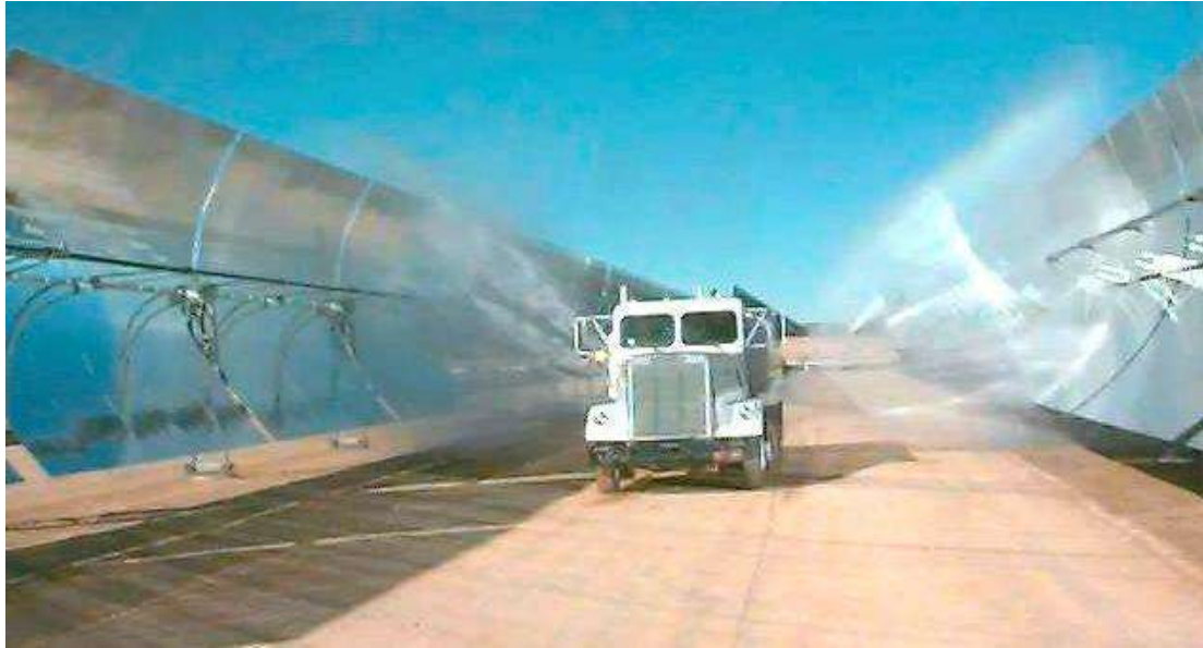
Figure 5-5: Trough reflector cleaning at SEGS
