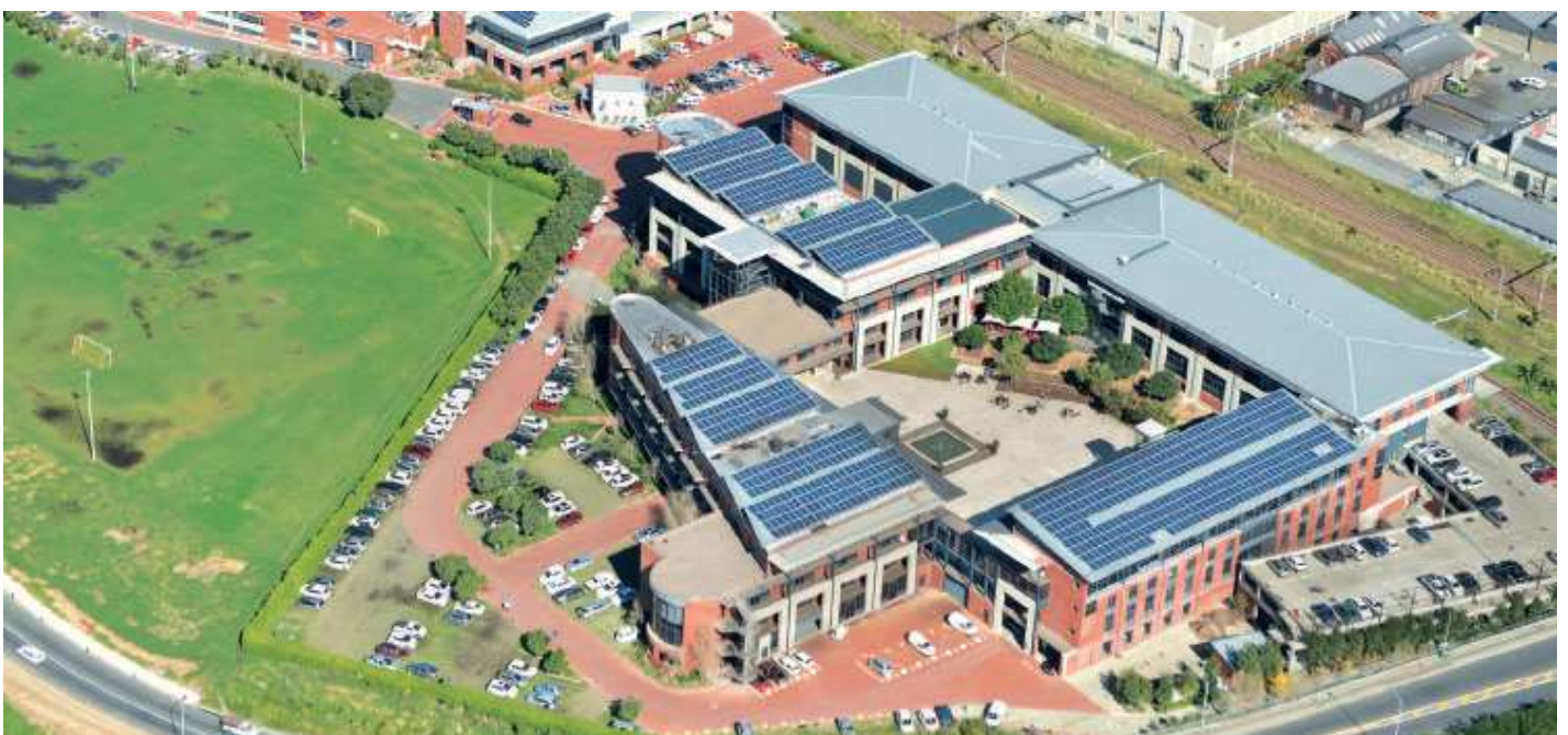
Grid-tied PV system at Black River Park.
